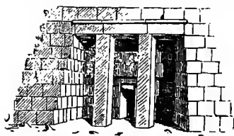
Fig. 123.—Portico and door, from Mariette's Les Mastabas .
